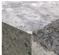
Steel fiber concrete
