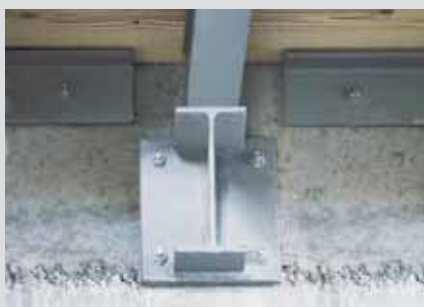
Fixing of steel beams, consoles and handrails
