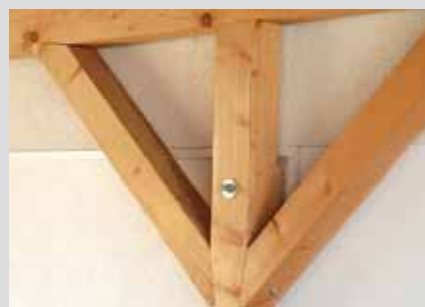
Fixing of timber structures
